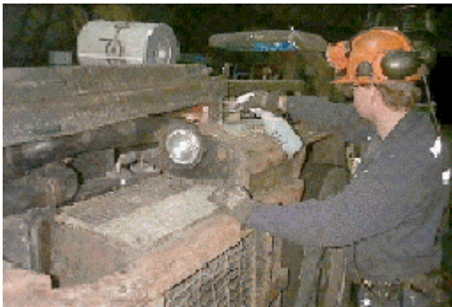
Fig. 7-5 Mechanic Testing an Intake System
