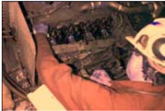
Fig. 8-17 Mechanic Servicing a Fuel System
