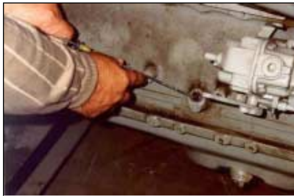
Fig. 11-1 Mechanic Checking Oil Level
