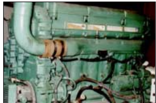
Fig. 3-3 Intake Manifold System
